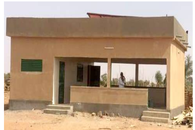
House of electricity services
