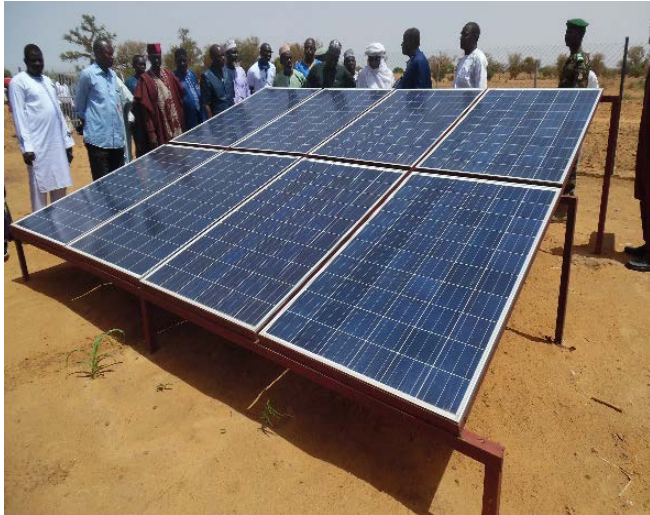
Park of solar panels
